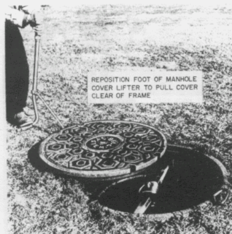
Fig. 33—Pulling Cover Clear of Frame
