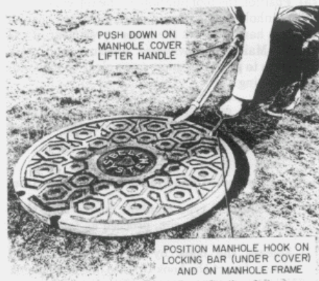
Fig. 32—Positioning Manhole Cover Hook on Locking Bar and Manhole Frame
