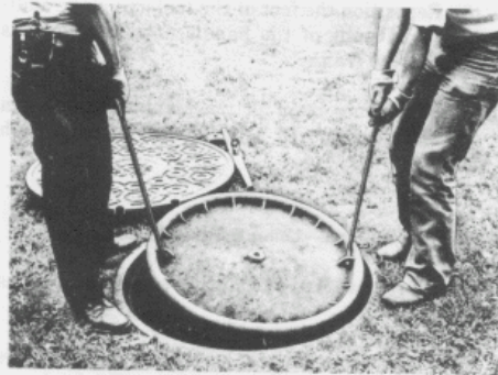
Fig. 38—Removing Inner Cover—Two-Person Method
