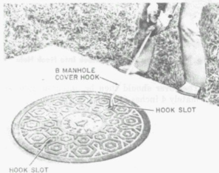
Fig. 12 -- Preparing to Unseat Type R Manhole Cover
