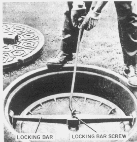
Fig. 27—Loosening Locking Bar Screw
