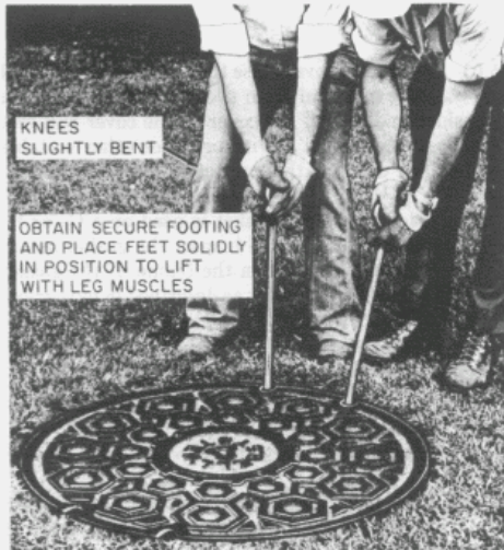
Fig. 34—¶Preparing to Unseat Cover—Two-Person Method¶
