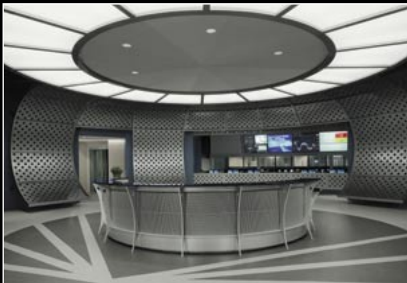
Convergent's reception area, looking into the network operations center designed and installed by BC Group.
