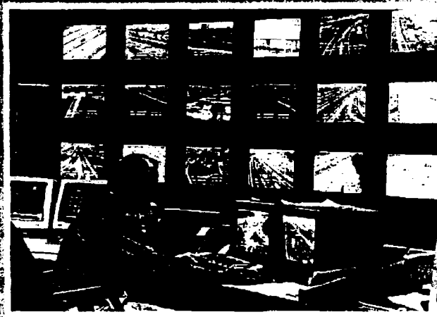
Central Monitoring Stations
