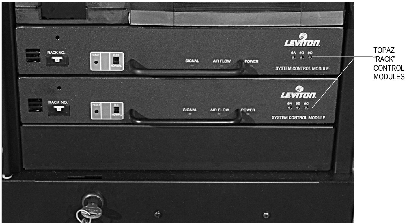
Figure 7 – Control Module Installation
