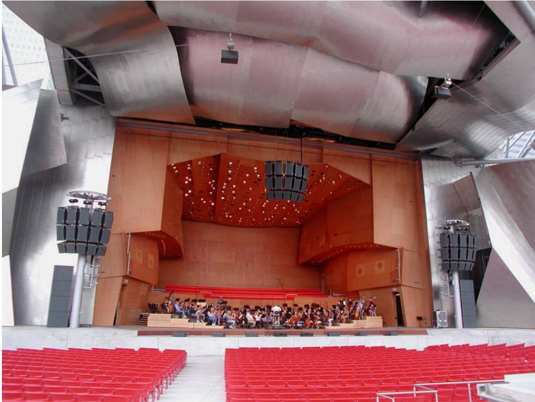
Figure One: EV® X-Array™ LCR reinforcement system covering the fixed seating area
