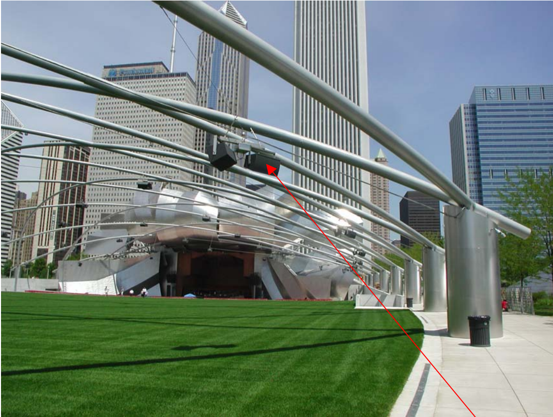
Figure Two: View from edge of lawn. The in-firing speaker is a Frazier custom cabinet for the enhancement system. The right-firing speaker in this photo is an EV Xi-1123A/106F full-range.
