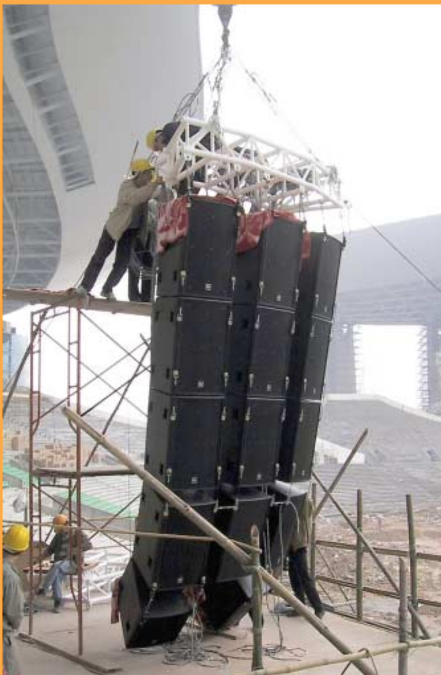
Workers at the Olympic Stadium in Beijing, China, prepare to hoist a massive X-Array cluster into place during construction of the stadium.
