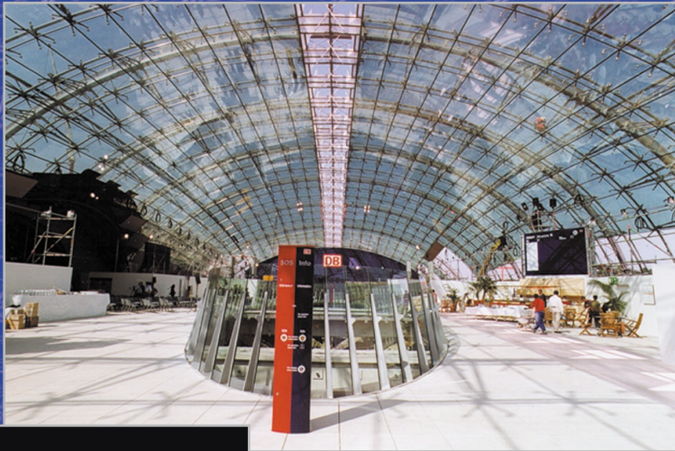
AIRFLY STATION FRANKFURT
