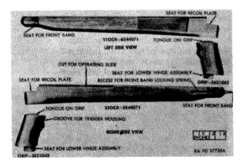
Figure 106. Stock and grip for carbine M1A1.
