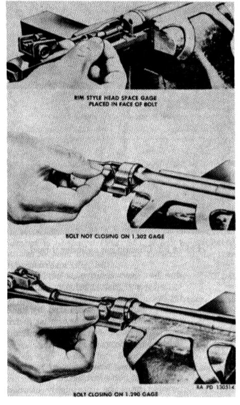
Figure 82. Checking head space.
