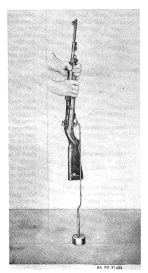
Figure 43c. Testing trigger pull.
