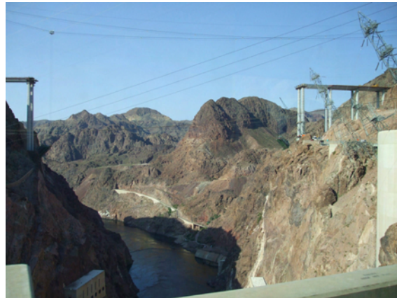
Top: Hoover Dam from the east side Lower: Part-built bridge (held up by a redesign: original thought to be at risk in high winds; completion now due 2010)
